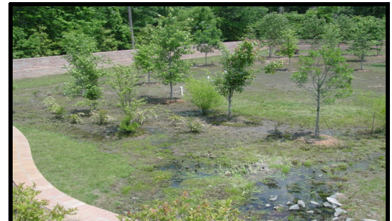
Structural stormwater controls, like this bioretention cell, may become commonplace in new Hillsborough developments.
