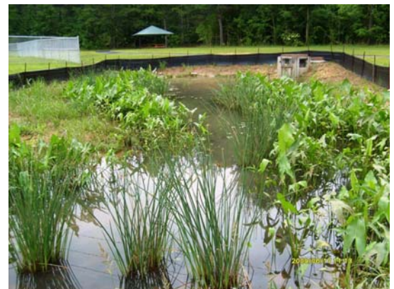
Stormwater wetland about one month after the initial planting.
