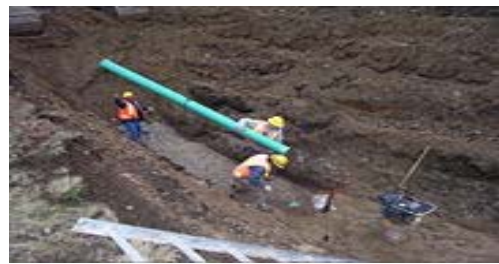
New sewer main installation
