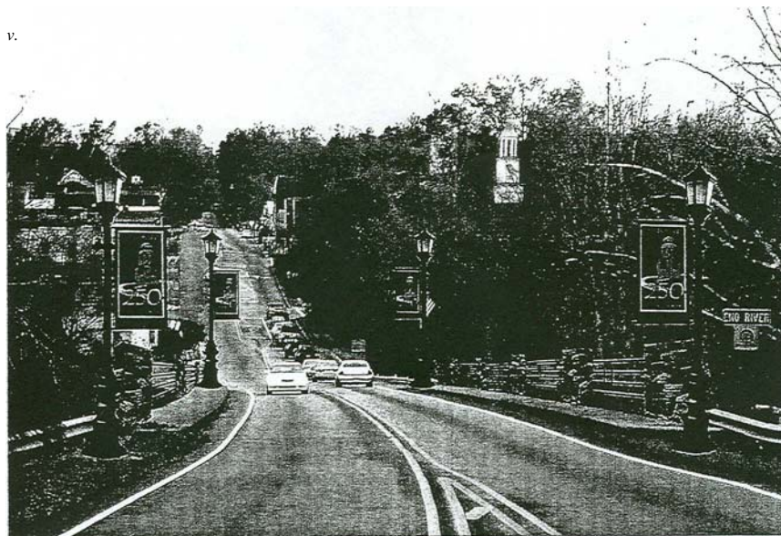
Figure 6. Eno River Bridge with new railings
